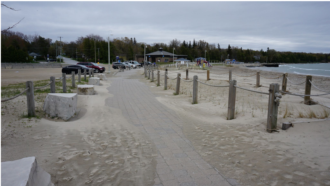
Figure 2 – Aeolian Transport of Sand Over the Walkway in Port Elgin (April 30, 2021)
