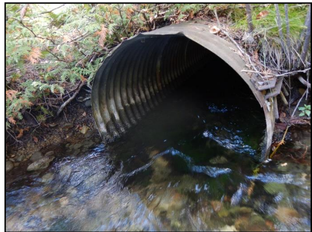
Photo 4 – Control Structure, Downstream
