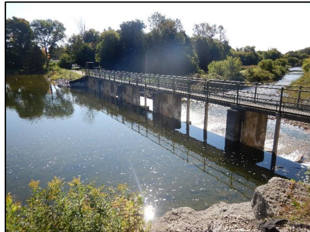
Photo 2 – Control Structure, Upstream
