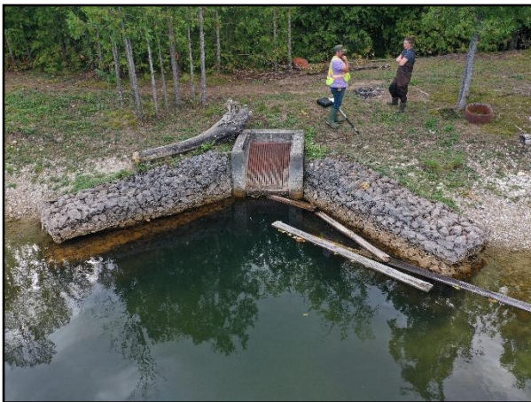
Photo 3 – Control Structure, Upstream
