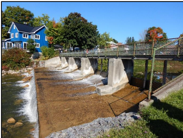
Photo 3 – Control Structure, Downstream
