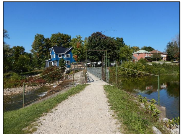
Photo 16 – Fencing along the Left Wingwalls
