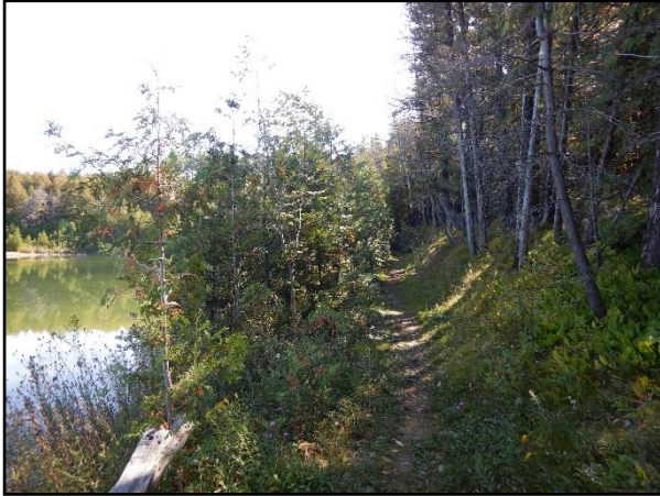
Photo 5 – Left Earth Embankment
