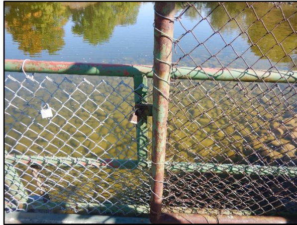
Photo 17 – Lock Securing Gate on the Structure Deck
