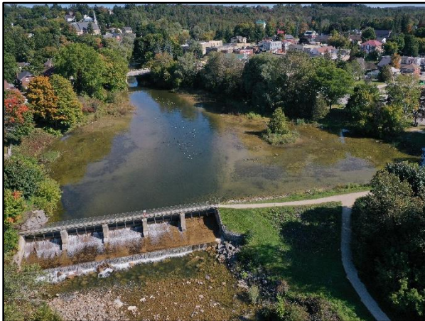
Photo 1 – Access Trail, East Side of Dam
