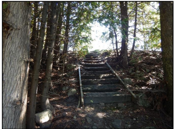
Photo 8 – Access Stairway on Downstream Side of Earth Embankment
