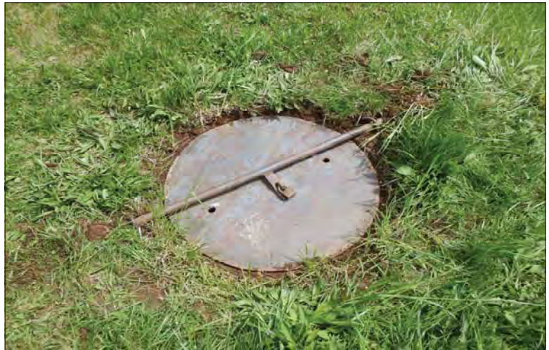
Filename: DSCN8064.JPG Photo 106 - May 15, 2024 Durham Upper Dam and Dyke Manhole Structure in Dyke
