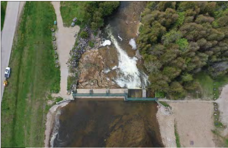
Filename: DJI_0692.JPG Photo 83 - May 15, 2024 Durham Upper Dam and Dyke Overhead View of Dam
