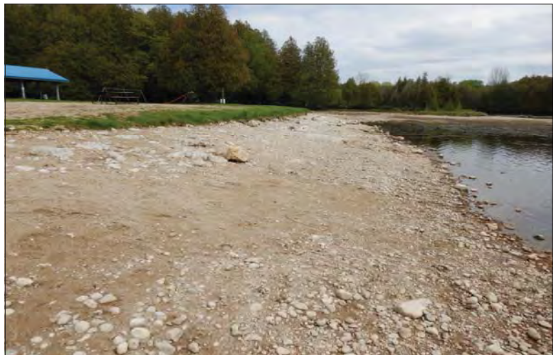
Filename: DSCN8033.JPG Photo 34 - May 15, 2024 Durham Upper Dam and Dyke Upstream Left Bank
