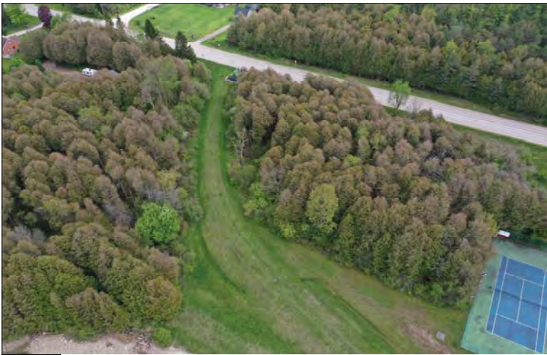
Filename: DJI_0688.JPG Photo 97 - May 15, 2024 Durham Upper Dam and Dyke Aerial View of Dyke
