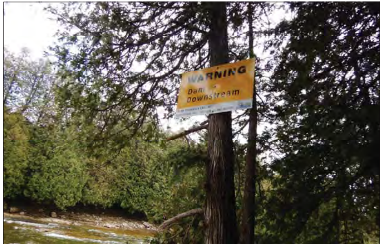
Filename: DSCN8093.JPG Photo 114 - May 15, 2024 Durham Upper Dam and Dyke Warning Sign Upstream of Dam
