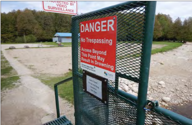
Filename: DSCN8015.JPG Photo 87 - May 15, 2024 Durham Upper Dam and Dyke Left Pedestrian Walkway Gate
