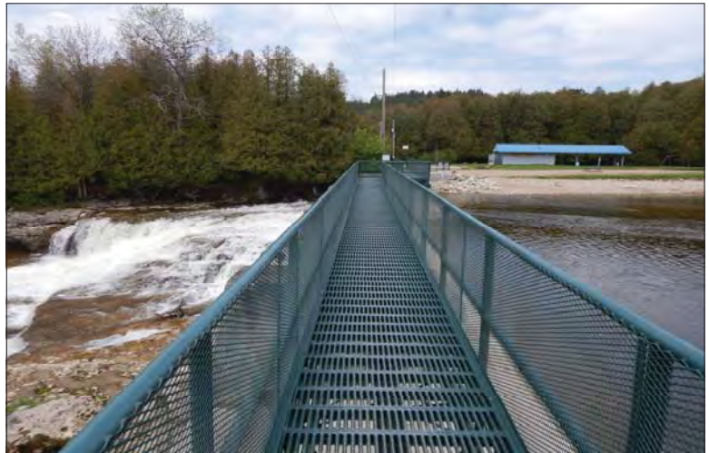
Filename: DSCN8005.JPG Photo 82 - May 15, 2024 Durham Upper Dam and Dyke Pedestrian Walkway
