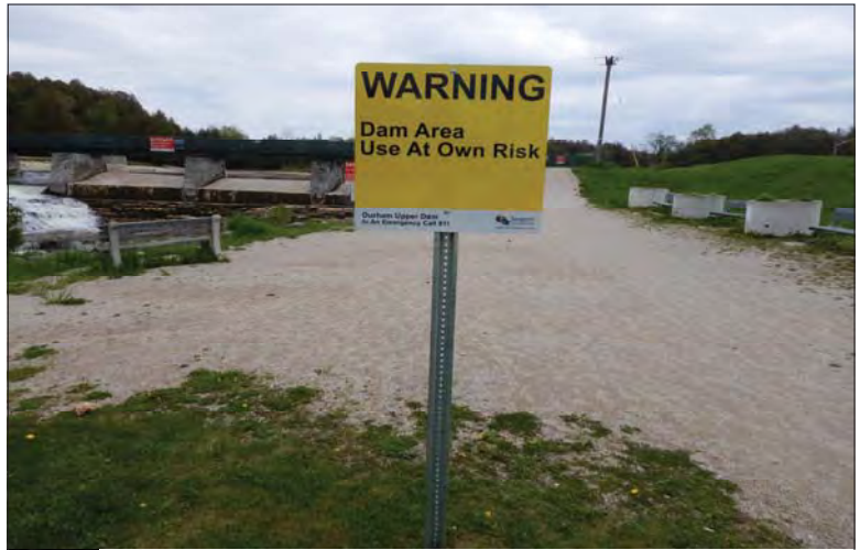
Filename: DSCN7915.JPG Photo 72 - May 15, 2024 Durham Upper Dam and Dyke Public Safety Sign on Downstream Right Side
