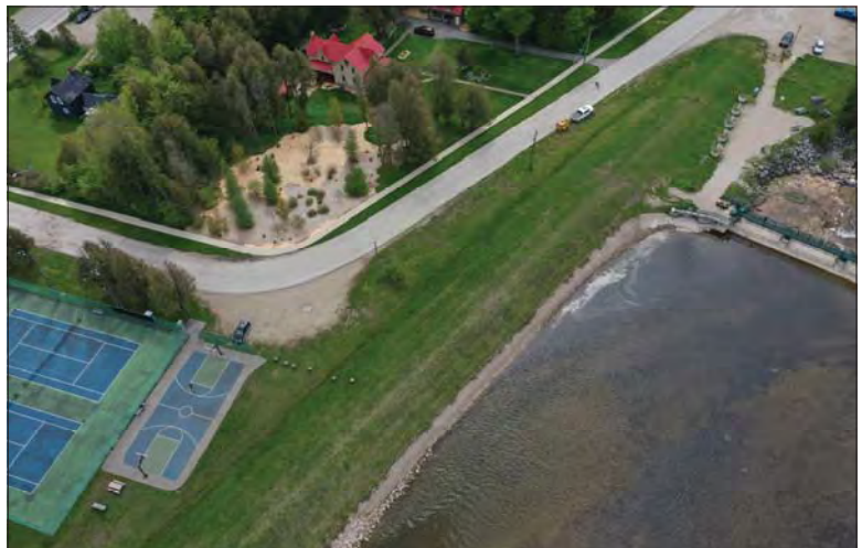
Filename: DJI_0690.JPG Photo 96 - May 15, 2024 Durham Upper Dam and Dyke Aerial View of Dyke
