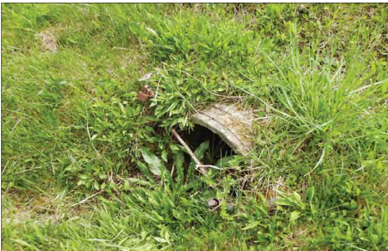
Filename: DSCN8062.JPG Photo 107 - May 15, 2024 Durham Upper Dam and Dyke Outlet Pipe
