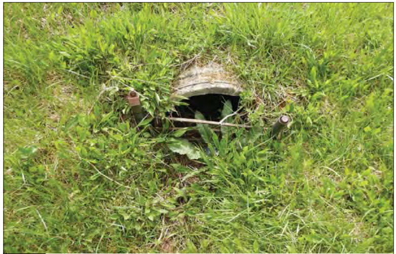
Filename: DSCN8057.JPG Photo 104 - May 15, 2024 Durham Upper Dam and Dyke Outlet Pipe
