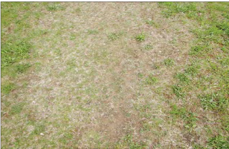
Filename: DSCN8047.JPG Photo 101 - May 15, 2024 Durham Upper Dam and Dyke Exposed Soil on Crest of Dyke
