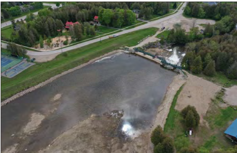
Filename: DJI_0684.JPG Photo 95 - May 15, 2024 Durham Upper Dam and Dyke Aerial View of Upstream Side of Dam
