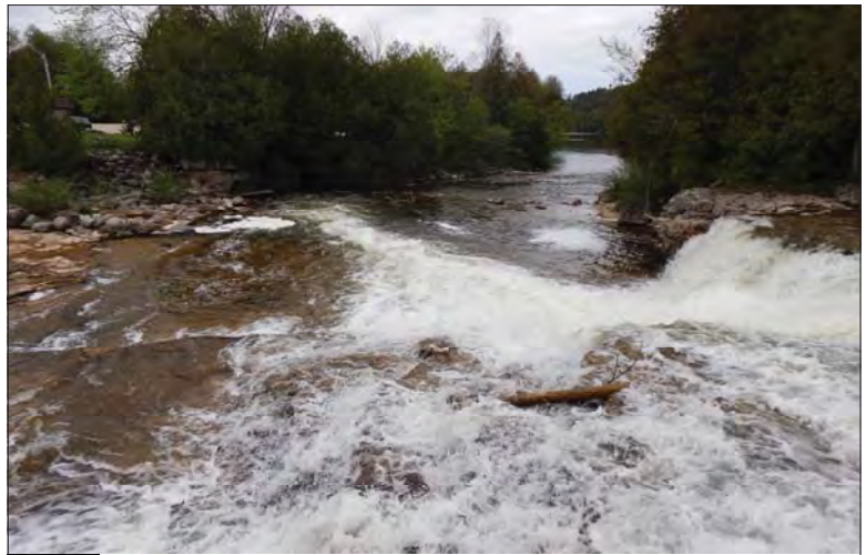
Filename: DSCN7981.JPG Photo 32 - May 15, 2024 Durham Upper Dam and Dyke Downstream Watercourse
