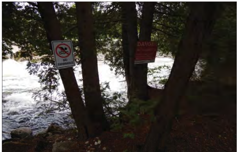
Filename: DSCN8094.JPG Photo 28 - May 15, 2024 Durham Upper Dam and Dyke Left Facing Public Safety Signs on Downstream Side
