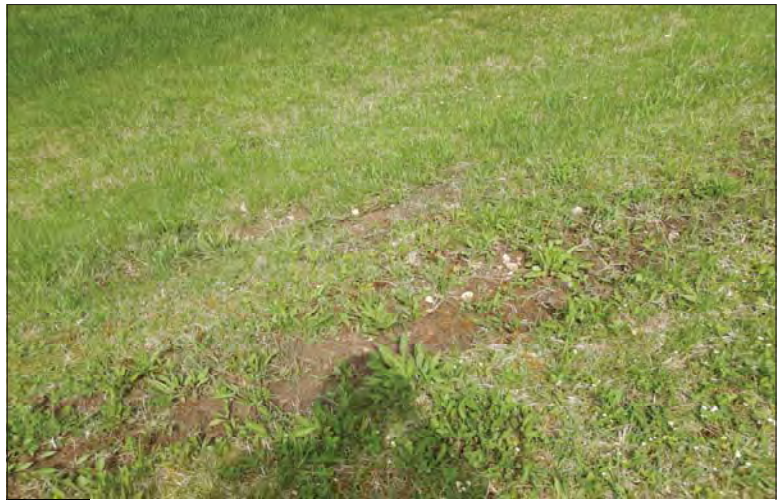
Filename: DSCN8066.JPG Photo 110 - May 15, 2024 Durham Upper Dam and Dyke Exposed Soil on Right Side of Dyke
