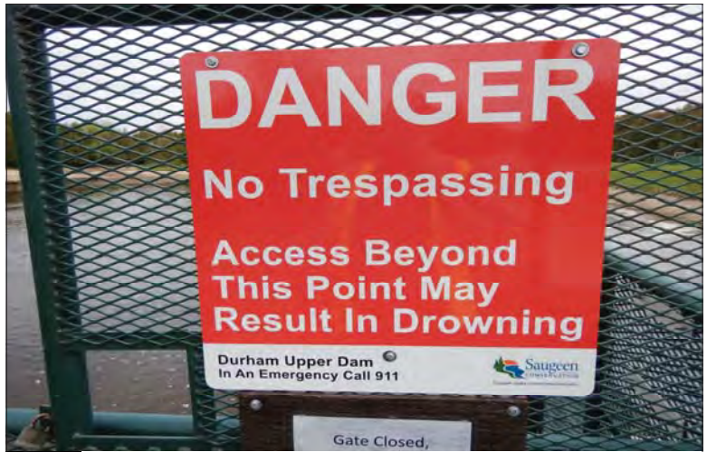
Filename: DSCN8002.JPG Photo 80 - May 15, 2024 Durham Upper Dam and Dyke Right Facing Public Safety Sign
