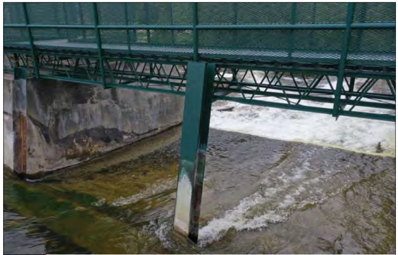
Filename: DJI_0656.JPG Photo 44 - May 15, 2024 Durham Upper Dam and Dyke Stoplog Gain in Centre of Sluiceway 2
