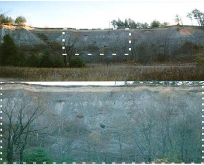
Figure 11 Piping erosion
